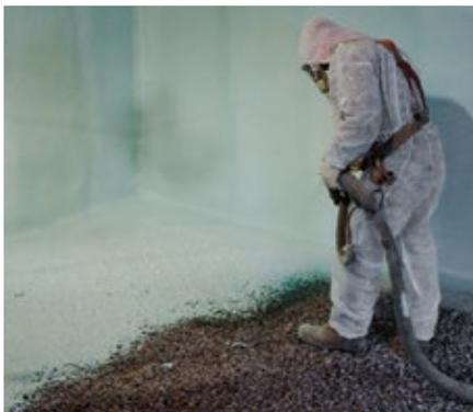
When a similar installation is done with the use of insulation panels, polyethylene, sealant, glue and tape, the overall performance and the quality of the job depend of the level of workmanship. In a single step with HEATLOK HFO Pro, we create a durable and perfectly sealed structural envelope during and after the work. All plumbing pipes and vents, sumps and drains in the slab and walls are sealed in one operation, without any complication regarding compatibility of materials.
